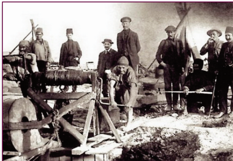
Circa 1895: Azerbaijani oil workers digging an oil well by hand in the Bibi-Heybat suburb of Baku.
